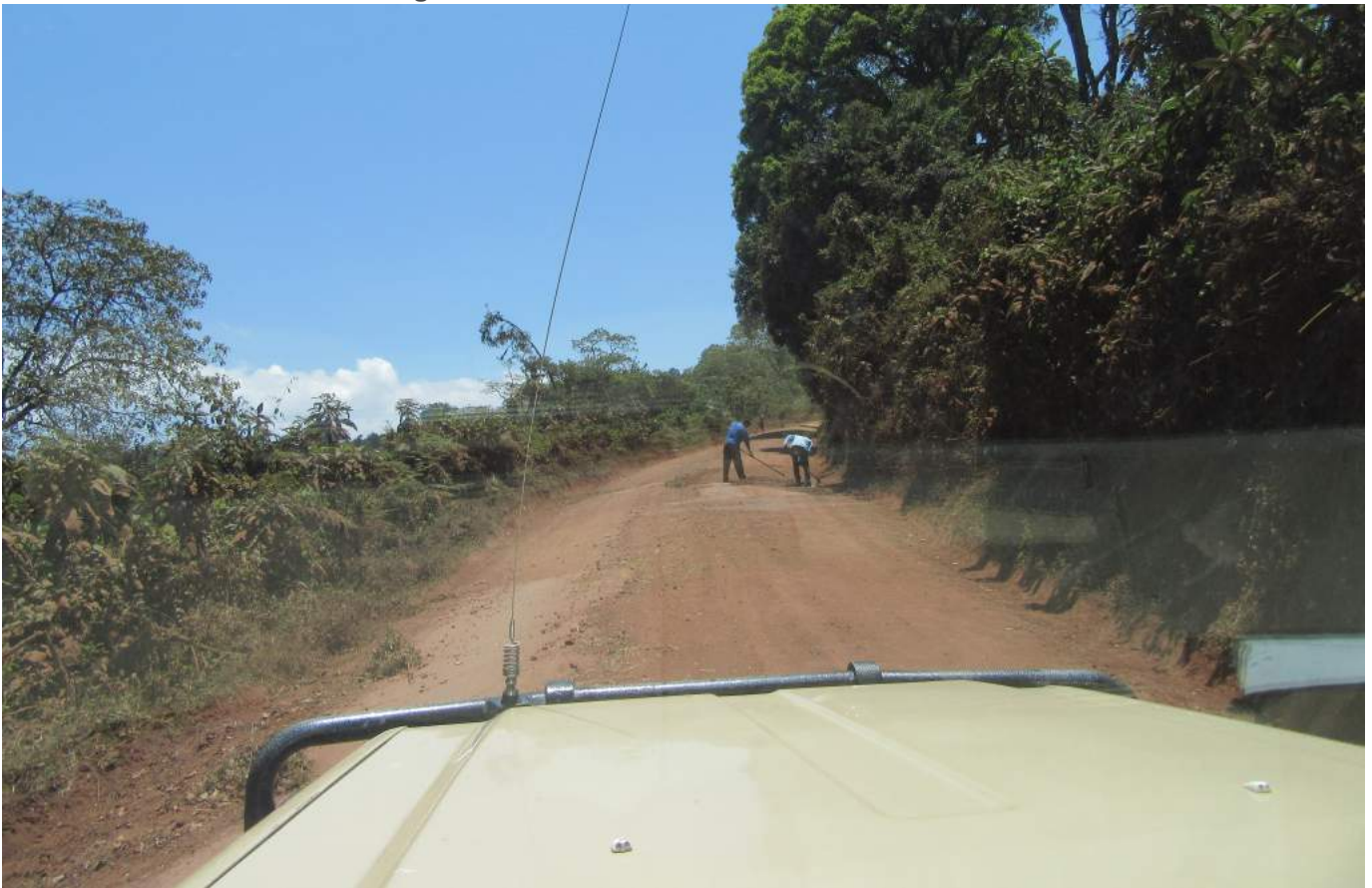
Workers maintain the road using hand tools.
